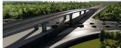
**Project:** The 10-kilometer road extension features 4–6 lanes, asphalt concrete pavement, two canal bridges, one overpass, and a drainage system to improve infrastructure and capacity.
